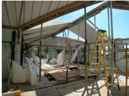
Insulating Concrete Forms Roof Structure, Walls & Floor Construction
