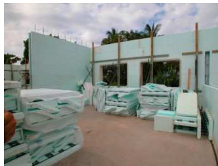
Insulating Concrete Forms Wall Construction, Note the Stacked Styrofoam Form Panels
