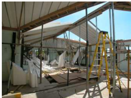
Insulating Concrete Forms Walls, Roofing and Flooring Construction
