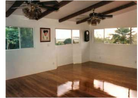
Living Room with New Hardwood Flooring, Stud Walls, Windows and Ceilings with Open Rafter Construction, Honolulu, Hawaii
