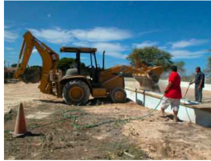
ICF Wall Construction, Backhoe Backfill Operations, Nanakuli, Hawaii
