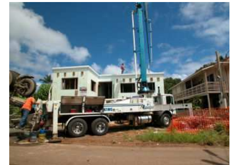
Concrete Grout Pumping Equipment, for ICF Home Construction on Flood Plain, Sunset Beach, N. Shore, Oahu
