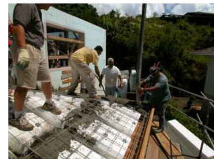
Insulating Concrete Forms, Three Story Home with ICF Walls, Floors & Hip Roofs, Makiki Heights, Honolulu, HI
