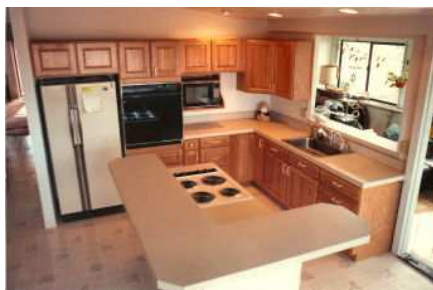
Complete Kitchen Remodel including New Cabinets, Counters, Flooring, Plumbing, Electrical, Sliding Doors and Windows, Kapolei, Hawaii
