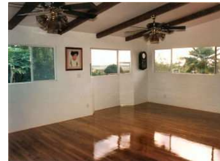
Living Room with New Hardwood Flooring, Stud Walls, Windows and Ceilings with Open Rafter Construction, Honolulu, Hawaii
