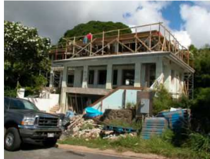
Construction of Three Story Insulated Concrete Forms Home, Makiki, Hawaii
