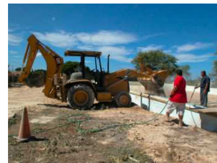
ICF Wall Construction, Backhoe Backfill Operations, Nanakuli, Hawaii
