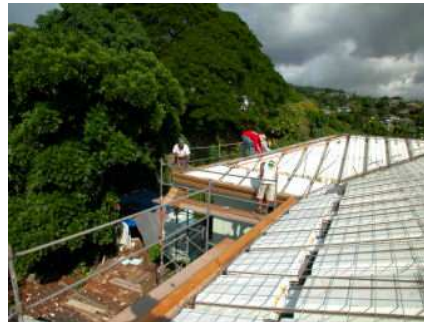
Innovative Construction of ICF Hip Roof with 4-12 Pitch
